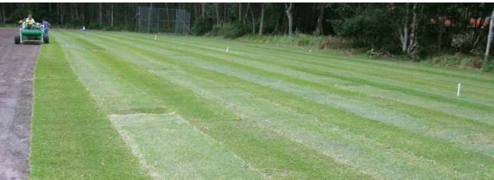
The turf goes down on a fully spec-compliant reconstruction.
