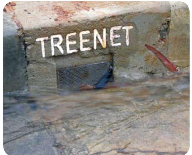
Treenet's Stormwater Inlet – a simple system to channel stormwater to trees planted into the verge. Put simply, water captured by the inlet fills a cubic metre, gravel-filled sump which then irrigates the surrounding beneath-pavement soil.
